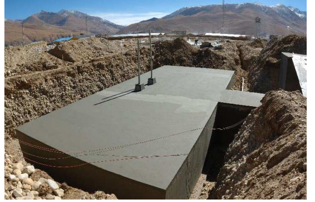
Fig. 10. Outside view of the prototype muon detector, which consists of two water cells, made of the reinforced concrete.
